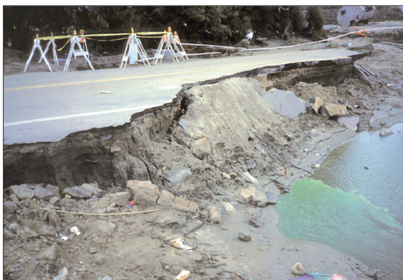
Figure 3. The Tijuana River flood in 1993 cut a new channel through the Tijuana River Valley, damaging Hollister Road, destroying an adjacent house, and moving sediment into the nearby estuary.
